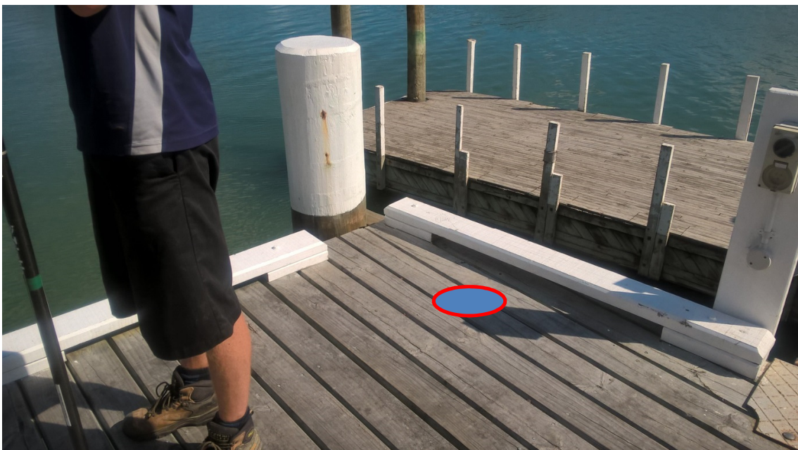
Figure 3. Shows proposed position for a “look-through” installation (blue and red circle, 120 mm diameter). The metal logger box will be placed over the hole as displayed in Fig 2 above.
