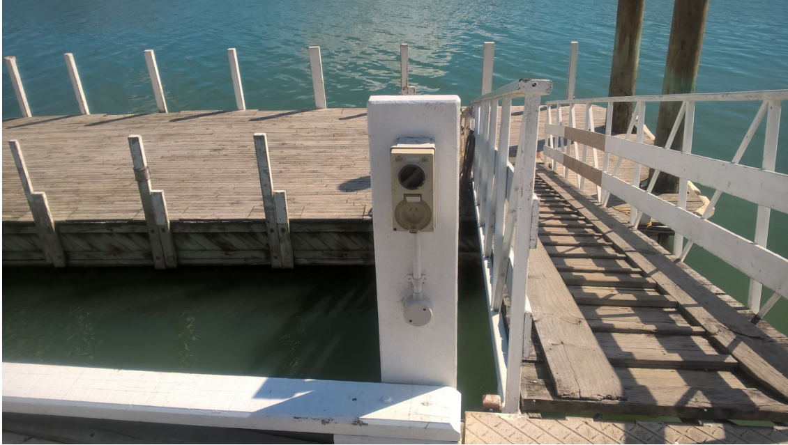
Figure 7. Power outlet adjacent to floating pontoon walkway
